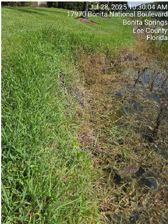
Lake 16 - Erosion needs repair.
